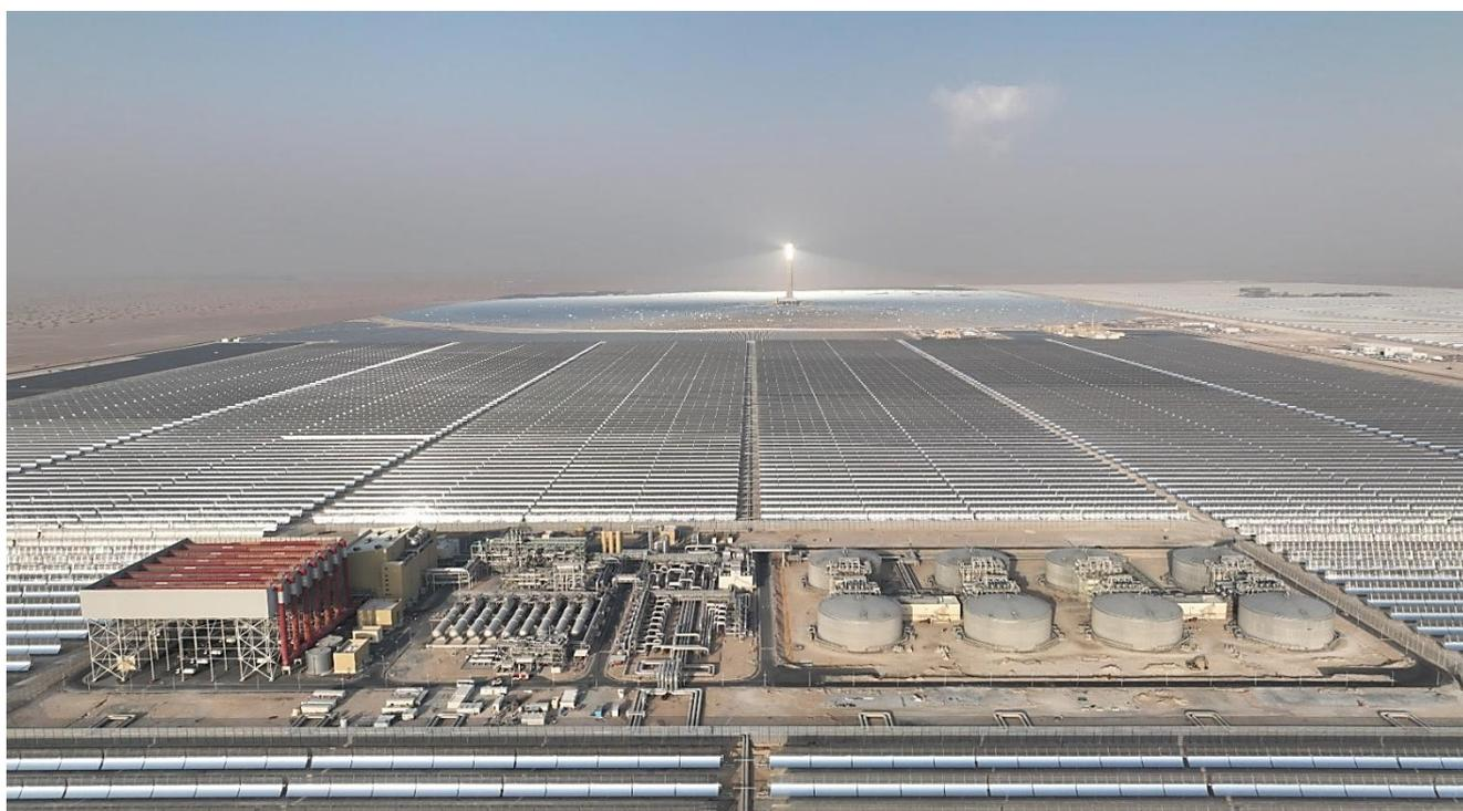
Construction project developed by the Company's EPC division, which includes three solar thermal plants with a capacity of 200 MW each in the "Mohammed bin Rashid Al Maktoum Solar Park" complex, the largest of its kind in the world. The project is located in Dubai, United Arab Emirates.
